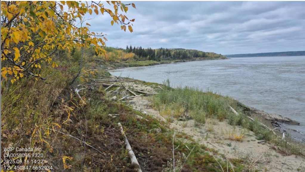
Photo 16 – toe of slope adjacent to the river showing erodible soils, high water marks, as well as tilted trees and scarps in the distance
