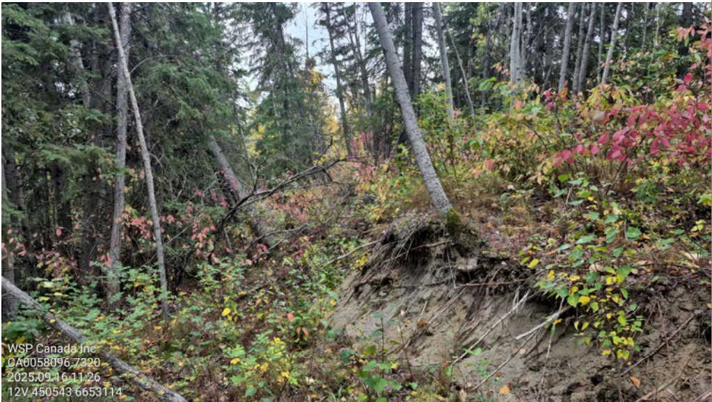
Photo 9 – area of fresh ground movement, torn vegetation mat and tilting trees/brush
