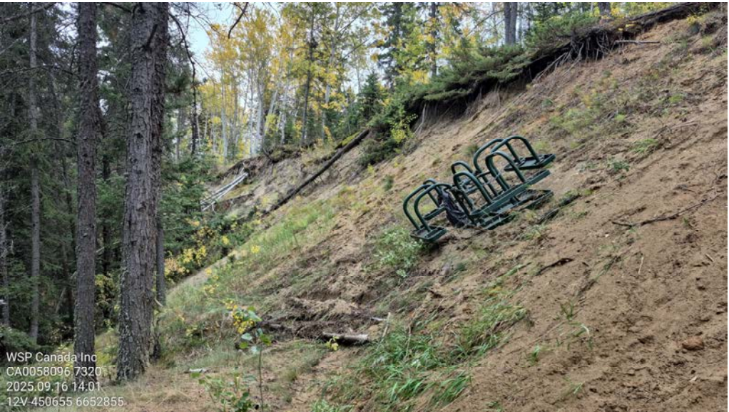
Photo 14 – headscarp, with overhanging j-trunk and fallen trees, overhanging vegetation. Vandalized picnic table in foreground.
