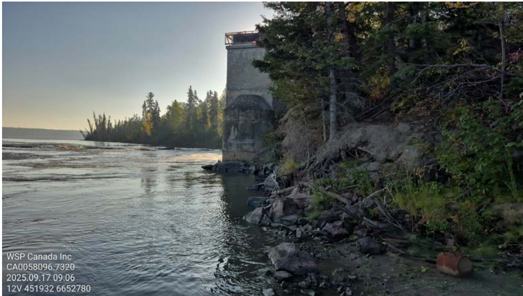
Photo 20 – water intake area. Note exposed suspected bedrock foundation and highwater mark
